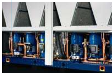
Optimised performance in the most common conditions thanks to multiscroll logic
